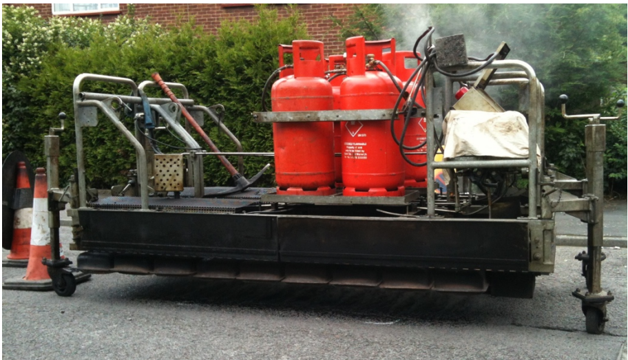
Figure 3. Picture of proprietary seam repair system.
